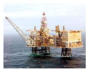
The DP platform comprises an eight-leg jacket supporting an integrated deck housing process train, gas treatment, flare boom, drilling facilities and derrick. The UQ platform comprises a four-leg jacket supporting an integrated deck housing utilities, living quarters, lifeboats, helideck, water injection, power generation and the exhaust structure.
