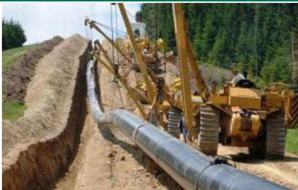
Positioning and lowering of a pipeline along an existing servitude/clearing through a wooded area
