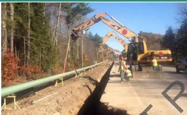
Positioning of a pipeline within a servitude using an existing road as access way
